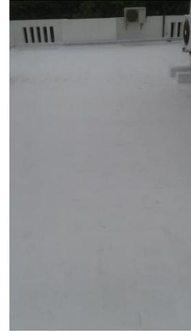
**At Karpagam Gardens Adayar in a flat of an area of 4000 sft the terrace was leaking. First terrace was cleaned and the at all tile joints and places where tiles were broken Featherplast was plastered. Then 2 coats of Surfapore thermodry mixed with exterior emulsion was applied.**
